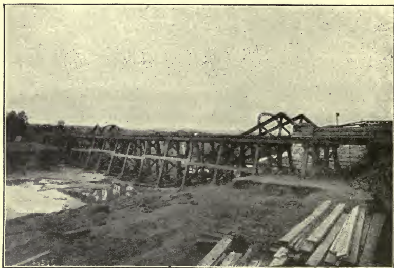
TEMPORARY BRIDGE AT FRERE.— Engineering.
