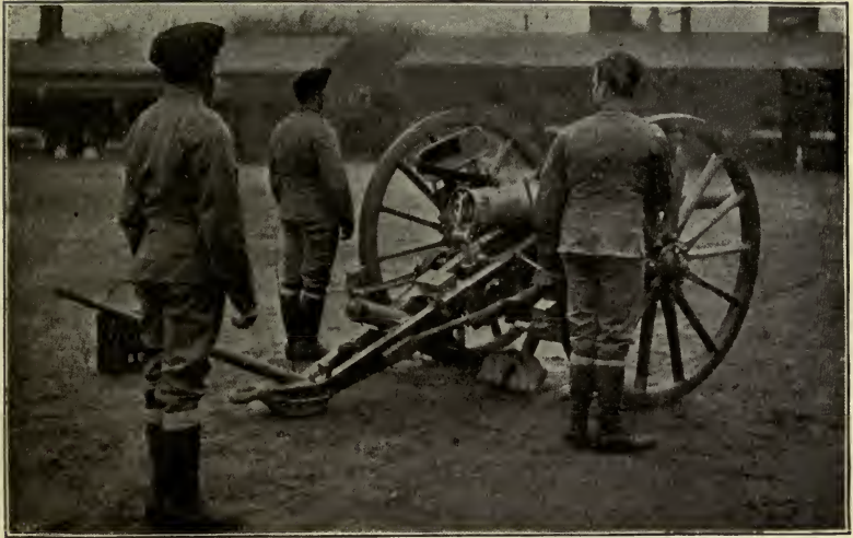
BRITISH FIELD GUN WITH CLARKE RECOIL BRAKE.
